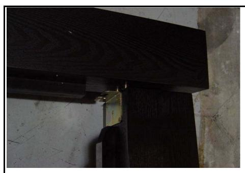
For the horizontal end there are two screws sticking out and for the vertical end there is a fixture that has two hooks looking thing.
